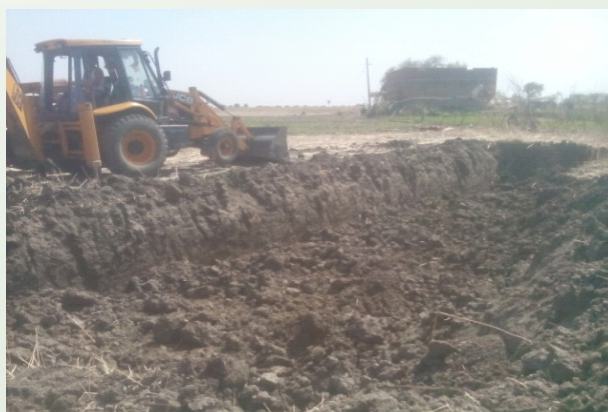
Excavation work in progress for construction of farm ponds in Nainwa block of Bundi district
