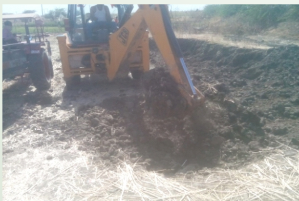
Excavation work in progress for construction of farm ponds in Nainwa block of Bundi district
